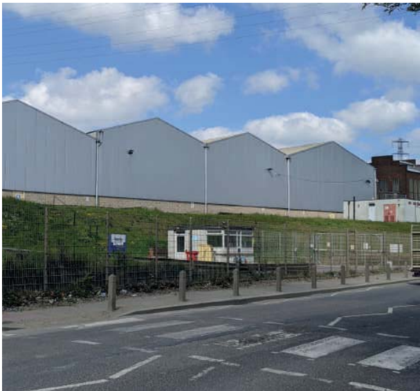
Figure 20: River Road looking North
