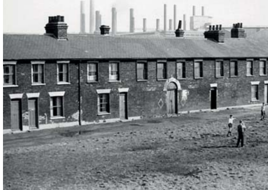
Figure 7: Creekmouth Village with Barking Power Station in background
