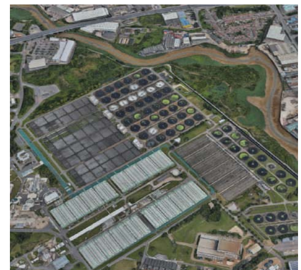
Figure 35: Beckton Sewage Works
