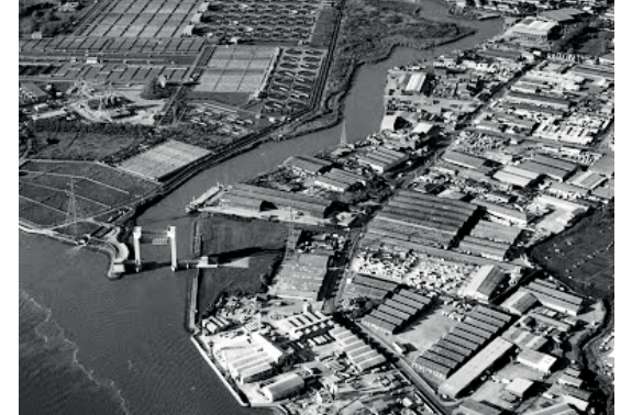
Figure 8: Aerial view showing Creekmouth Flood Barrier
